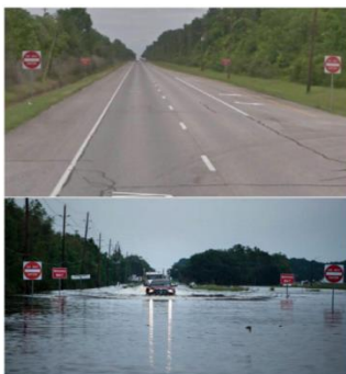
Figure 1: US 69 Before and After Flooding Resulting from the Impact of Hurricane Harvey
