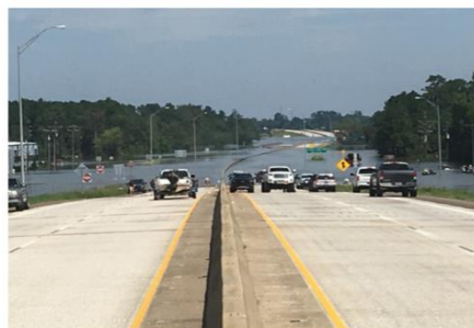
Figure 2: Flooded Section of US 69 from Hurricane Harvey Impacts
