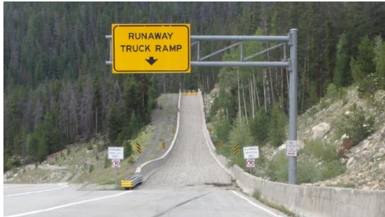
Figure 1: Colorado Loveland Pass confined ascending grade arrester bed EER
