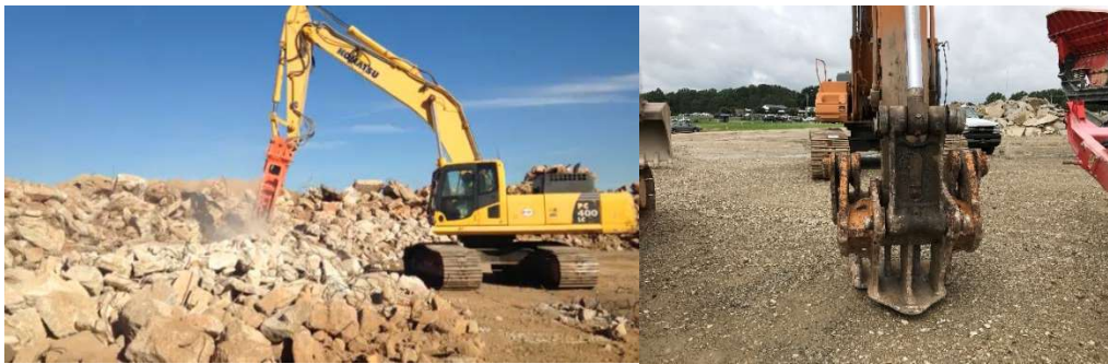
Figure 3: Concrete pulverizer used to size and remove concrete reinforcing steels – operation (left); jaw of the pulverizer (right).
