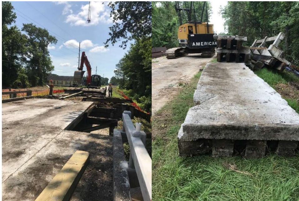
Figure 2: Concrete slabs removed - bridge where panels were removed in Beaufort County (left); panels removed from bridge in Sampson County, NC (right).
