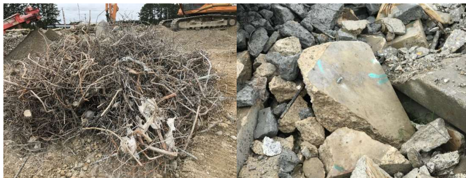
Figure 4: After pulverizing – most of reinforcing steel was removed (left); sized concrete for crushing and screening (right).
