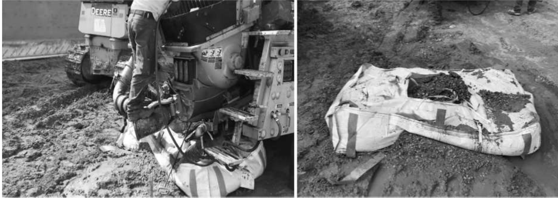
Figure 1 - Lined bag used to attempt washout containment, an unsuccessful norm
