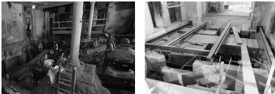
Figure 2: Below-slab micropile installation, ductwork and piping, March 2018
