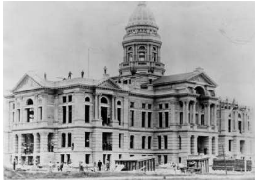
Figure 1: Wyoming State Capitol Construction, circa 1890, National Park Service .
