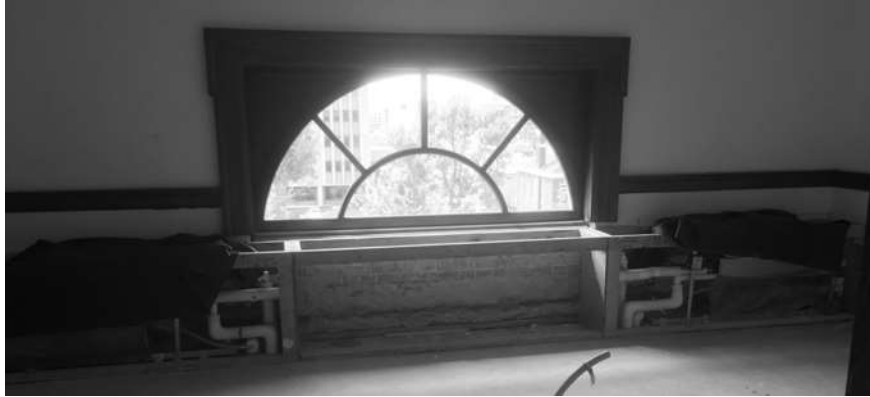
Figure 3: Fan coil units framed for built-in decorative woodwork.
