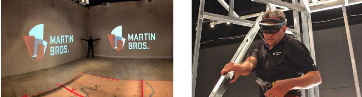
Figure 3: Use of HoloLens for building a bathroom pod using a hologram. (images courtesy Martin Bros., CA)
