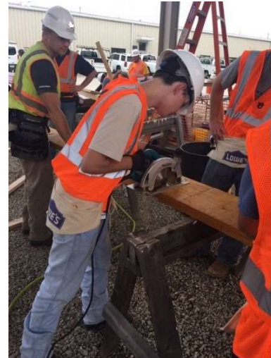
Figure 3: Camper Making Framing Cuts
