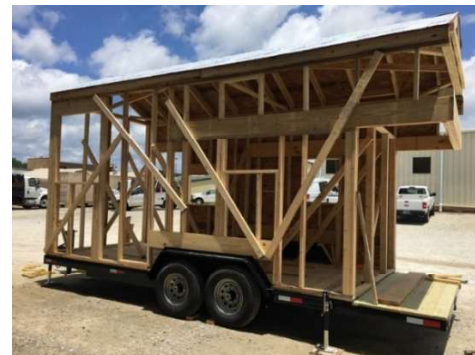
Figure 5: Project at the end of the camp
