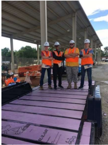
Figure 2: Trailer Insulation Complete
