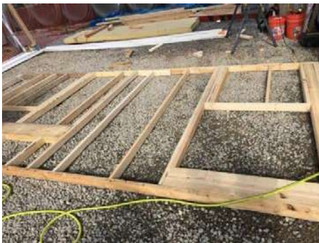
Figure 4: Framing for one Side (Long) Wall
