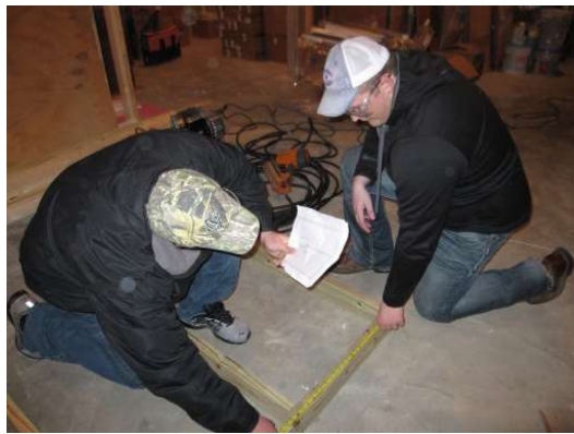
c. Fieldwork in finishing the basement of a green home
