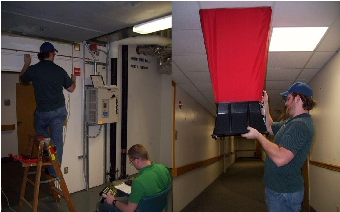
Figure 1: Duct traverse (left) and flow hood (right) airflow measurements (Grosskopf and Mousavi, 2014).
