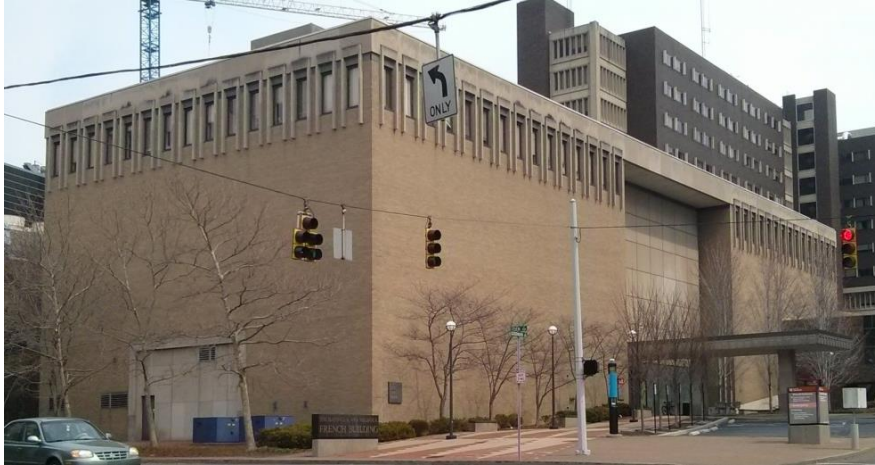
Figure 1: The building used in the case study (actual site photograph).
