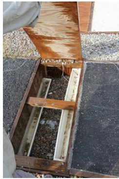
Figure 2: Collection gutters with plywood cover to protect from heat gain.
