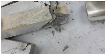
Figure 7: Beam shear failure type
