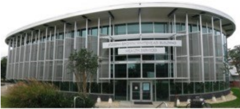
(a) Stamps Health Center building on XXXXXX campus
