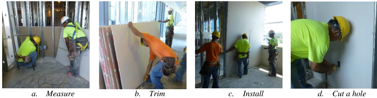
Figure 5: Conventional drywall installation procedure.
