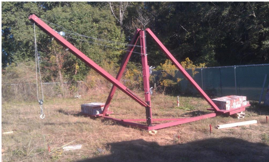
Figure 2 – Picture of completed Derrick Crane
