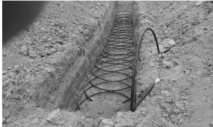
Photo 1: Flexible Pipe Slinky Placed in a Trench
