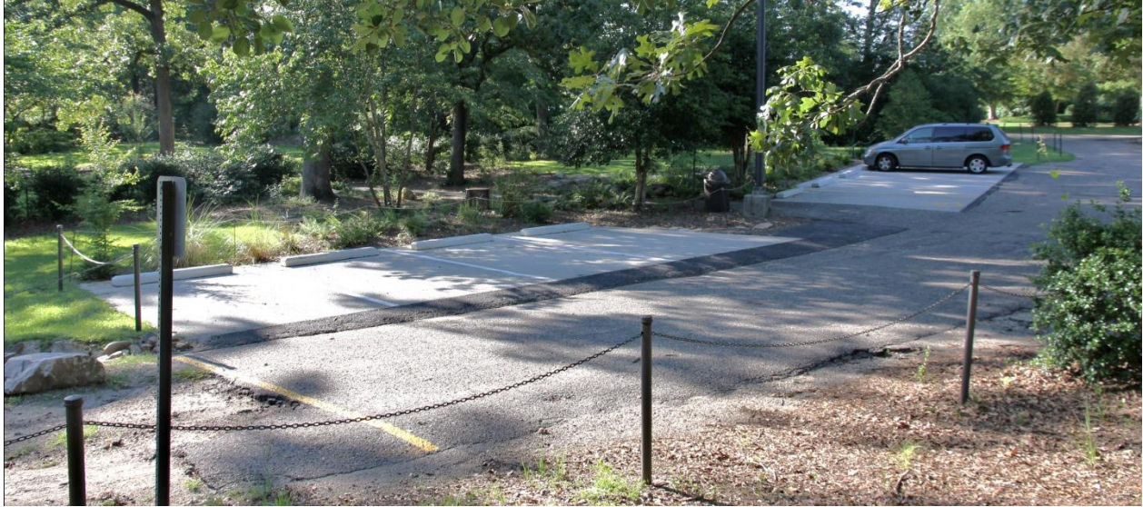
Figure 3: Completed PC paved parking lot.
