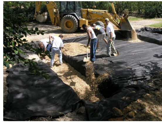
Figure 4b: Backfilling Cross Trenches with open graded gravel
