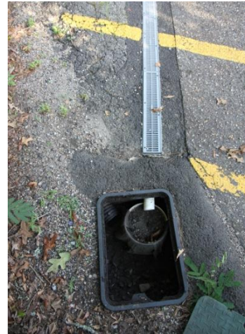
Figure 7b: Runoff collection reservoir
