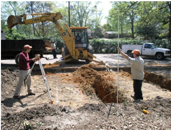
Figure 4a: Constructing Cross Trenches for captured stormwater storage
