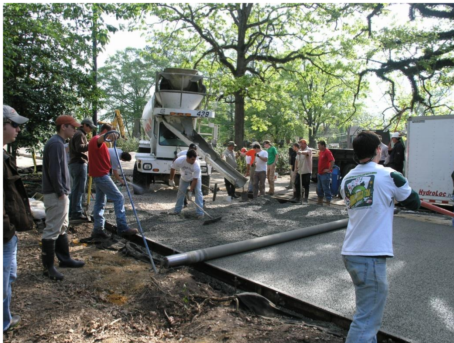
Figure 8: Students and university facilities workers place PC pavement with contractor
