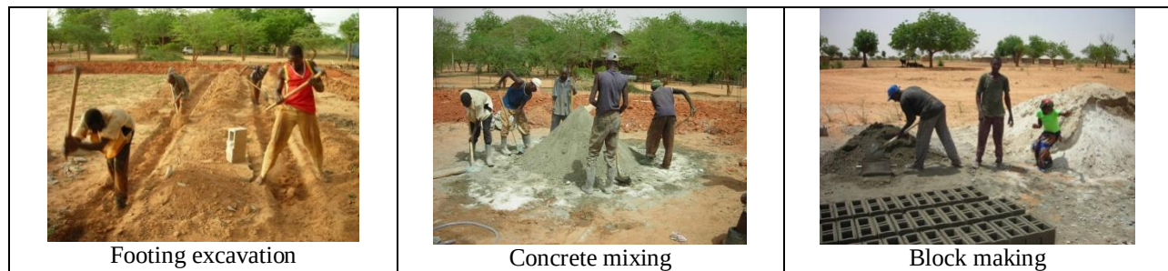
Figure 1: Developing World Construction Methods
