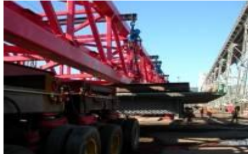
Figure 1: SPMTs transporting new deck panel from fabrication site adjacent to bridge.
