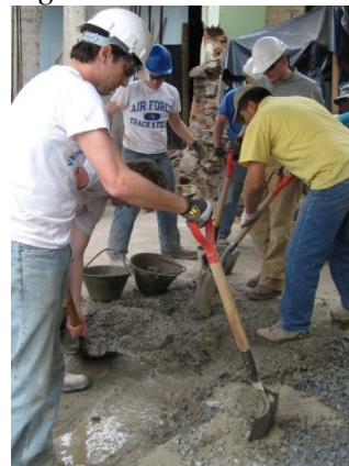
Figure 4: Mixing Concrete
