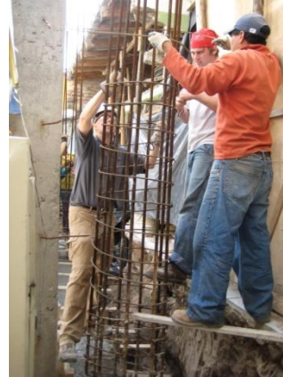
Figure 2: Column Rebar
