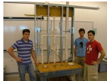
Figure 5: Students dry fit a drain, waste and vent system and plumb the potable water
