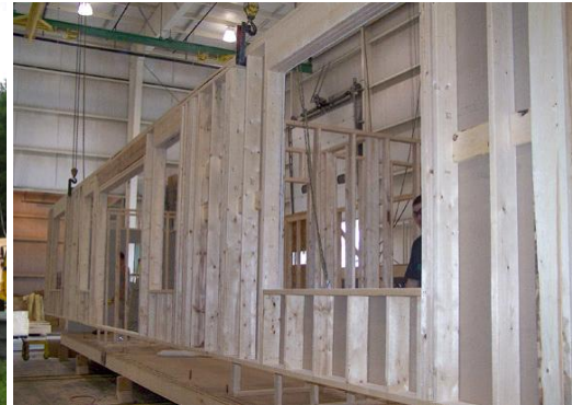
(c) Prefabricated Wall Panels
