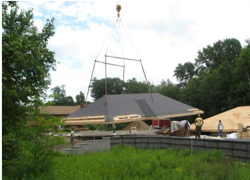
(b) Installation prefabricated Roofs
