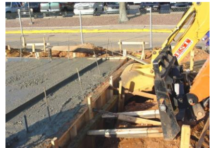
Figure 1c: The Machines Held the Frame up while the Concrete Set
