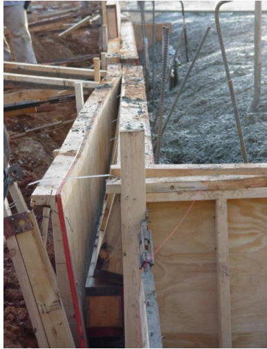
Figure 1a: The Frame Blew-out during the Pour
