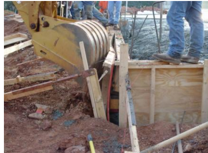
Figure 1b: The Backhoe-loader pushed the Frame Back Vertical to Hold Concrete
