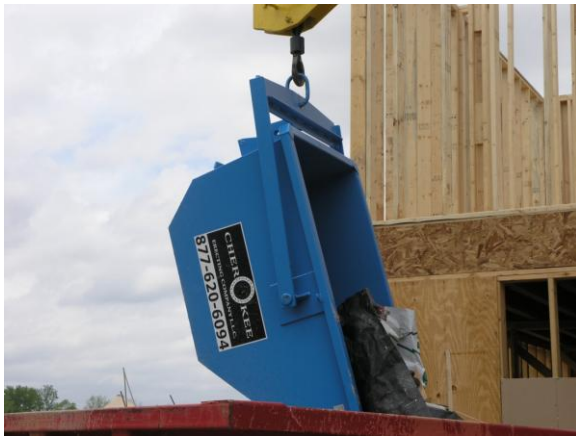
Figure 2: Self-Dumping Bins in Use on a Construction Site
