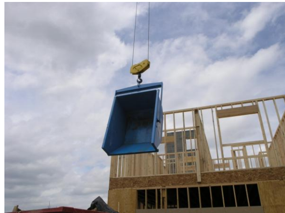
Figure 2: Self-Dumping Bins in Use on a Construction Site
