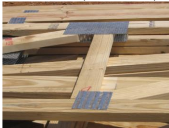
Figure 1: Metal plate connected wood truss
