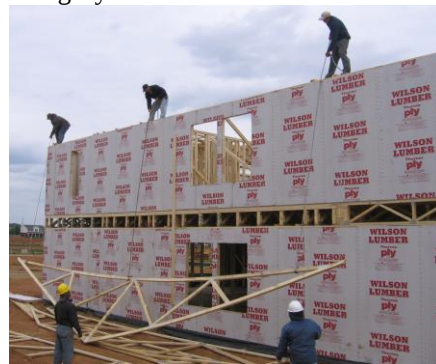
Figure 3: Lifting a truss by hand on a two story building showing lateral bending in truss.
