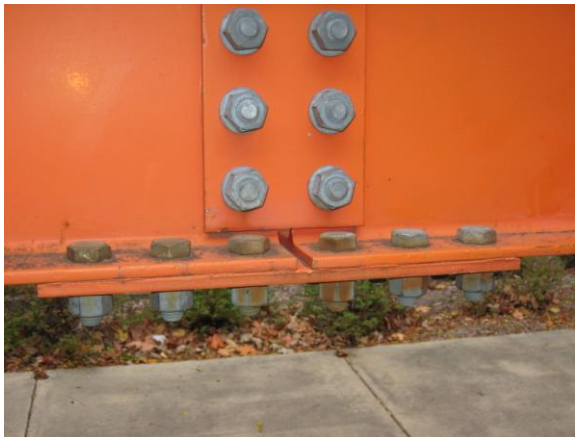
Figure 3: Photo and Detail of Steel Connection as Represented in Drawing for the North Elevation of AISC Steel Sculpture
