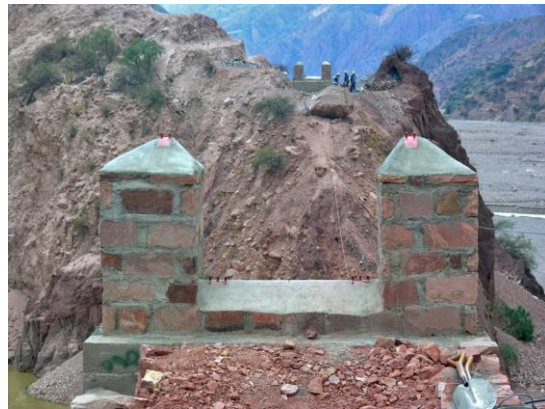
Figure 3: Close-up of Pedestrian Bridge Towers.
