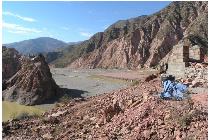
Figure 1: View of River Gorge with Bridge Tower on the right.
