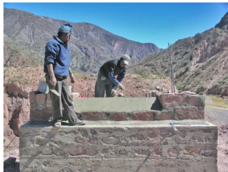
Figure 4: Local Villagers Helping Build Tower
