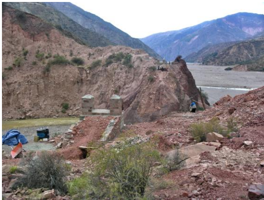
Figure 2: Pedestrian Bridge Towers and Span.
