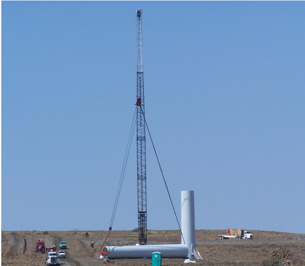
Figure 5: Erecting tower base with wheel-mounted crane.
