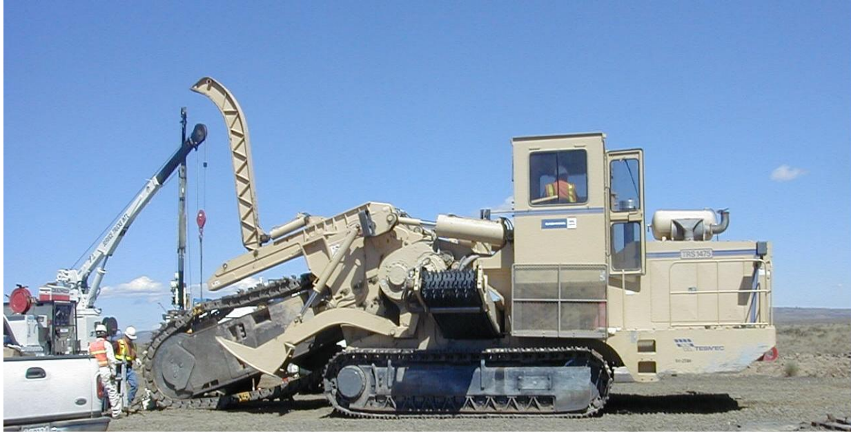
Figure 6: Maintaining the chain trenching machine.
