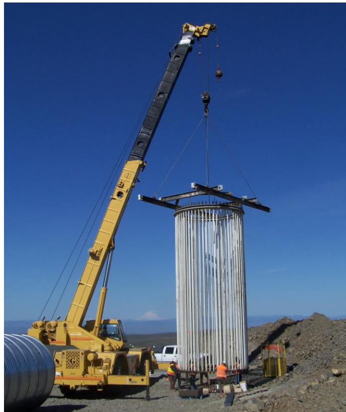
Figure 2: Lowering assembled bolt cage.
