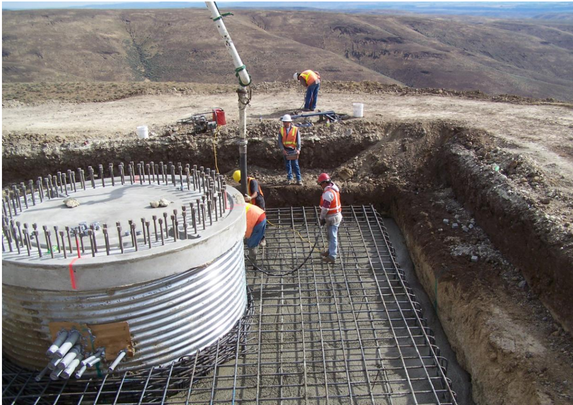
Figure 3: Pumping concrete collar around completed foundation in soft soil.
