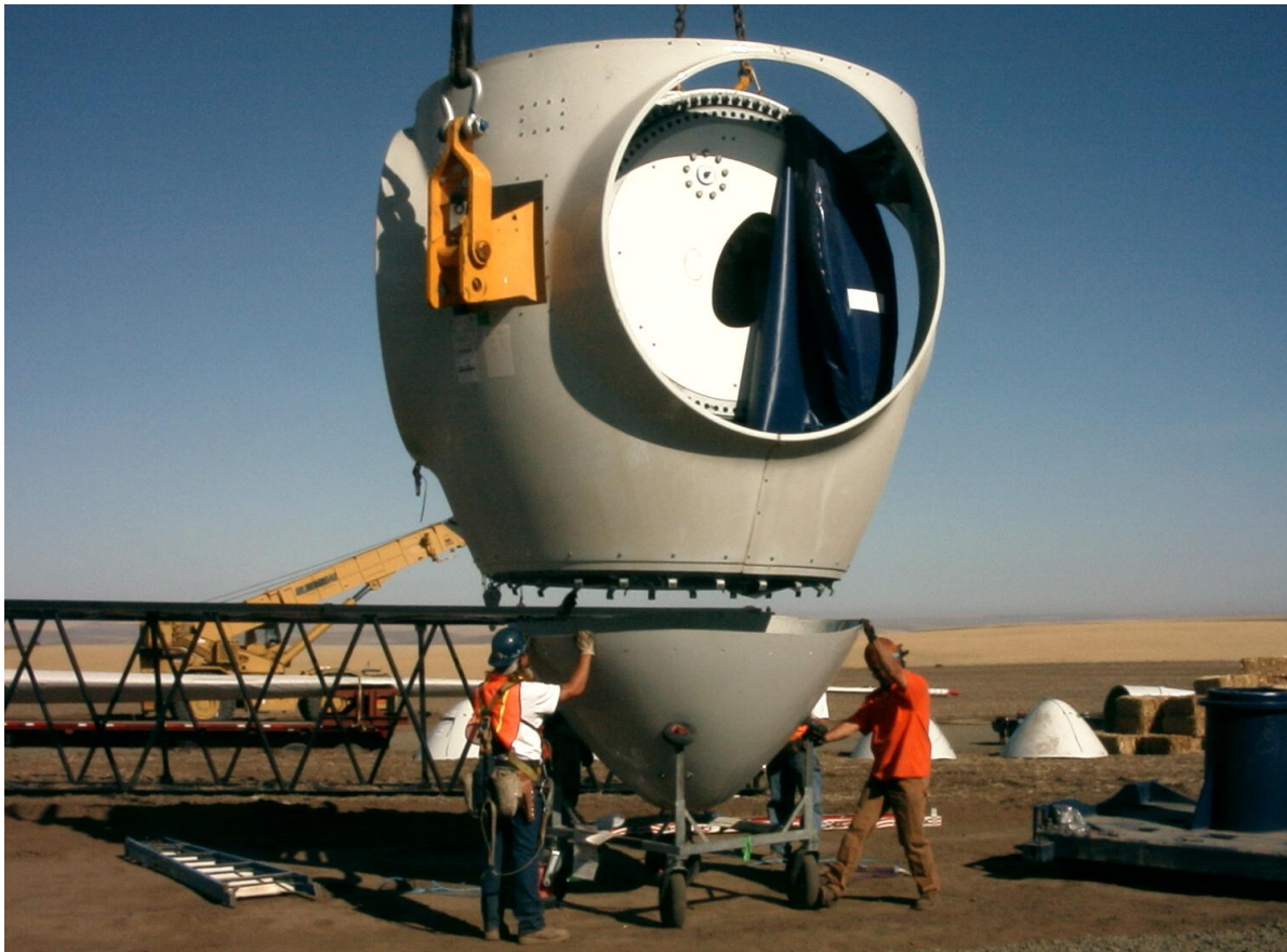
Figure 4. Assembly of nacelle in marshalling yard.
