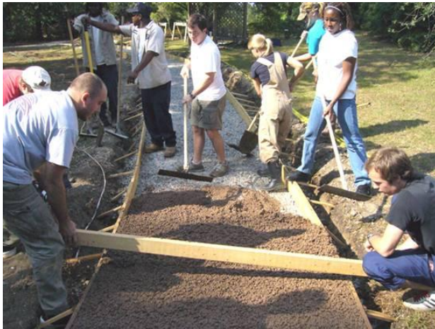
Figure 6. Deposit and strike-off
