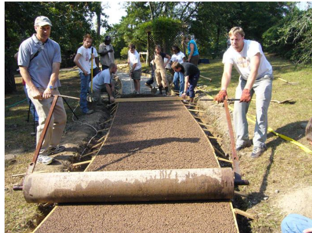
Figure 7. Compressing with roller
