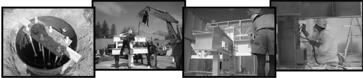
Figure 3: Footing form, erection, placement of painting enclosure, and applying final coating.
