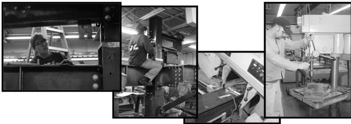
Figure 2: Welding students fabricating and erecting the SSTS.
