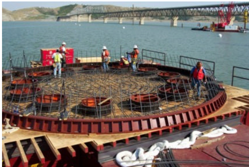
Figure 4: Pier 3 of the third Four Bears Bridge in 2004 (NDDOT, 2005)
