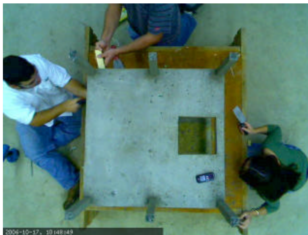
Figure 6: Stripping Second Floor Forms
