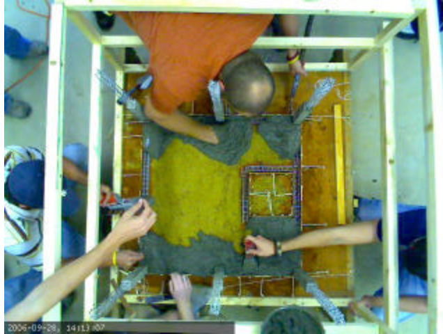
Figure 4: Placing the Slab On Grade
