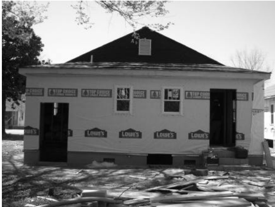
Fig. 6 - Completed Rear Addition
