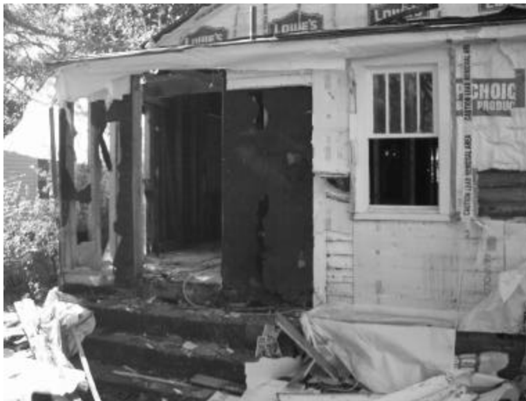
Fig. 5 - Rear Porch Demolition
