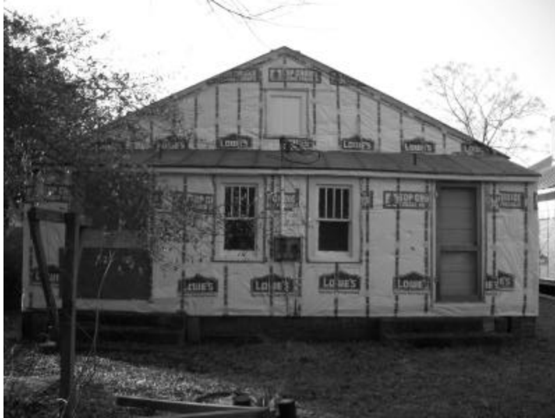
Fig. 4 - Existing Rear Porch
