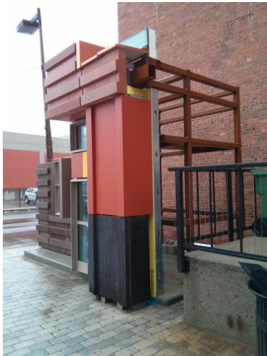
Figure 3: Physical facade mockup
